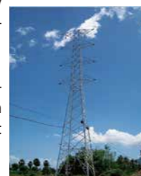
Power Transmission Tower
